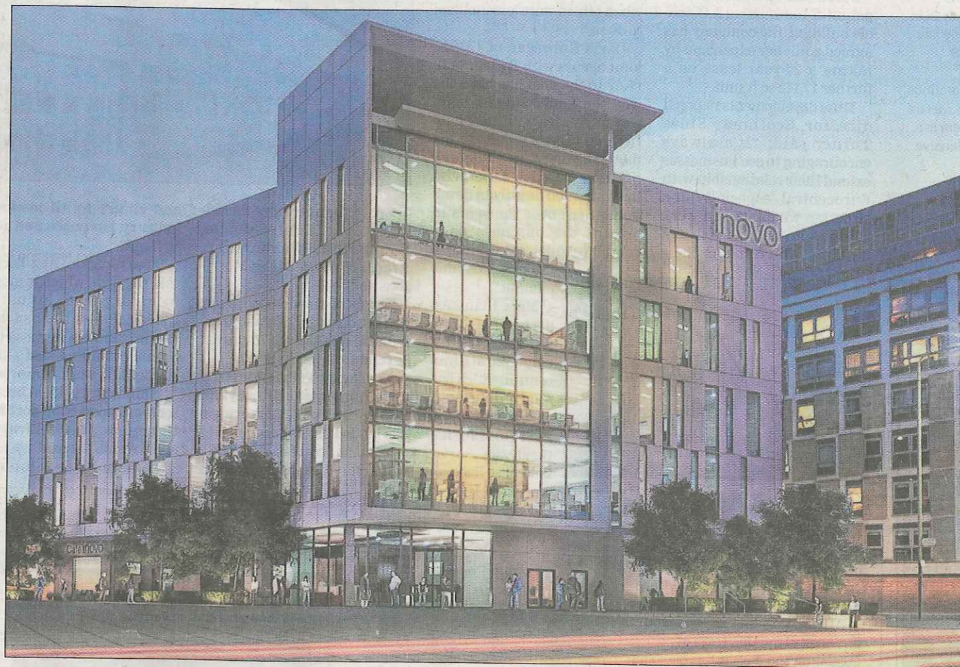
TOP MARKS: inovo has an 'excellent' efficiency rating and gets an A grade for energy performance.
